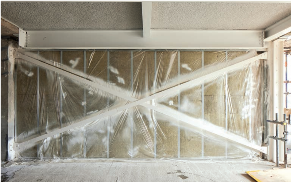
FIGURE 7: New steel cross-bracing installed at either end of building to provide additional stability
