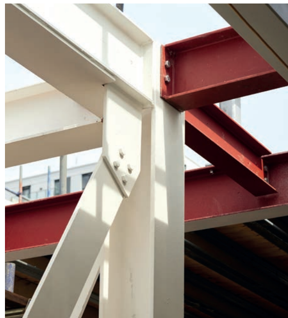
FIGURE 4: New steel framing at roof level
