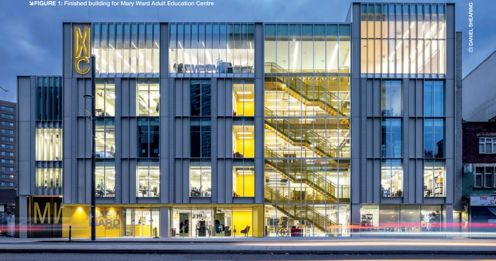
FIGURE 1: Finished building for Mary Ward Adult Education Centre
