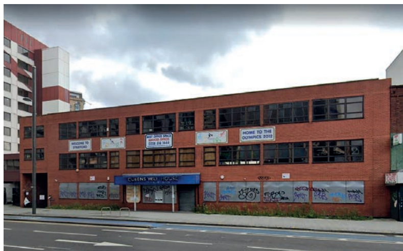
FIGURE 2: Queensway House (front elevation), pre-intervention
