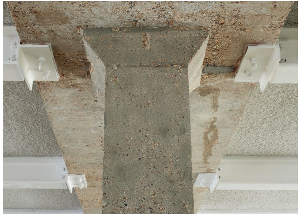
FIGURE 3: Concrete repairs and new steelwork to support additional upper storeys
