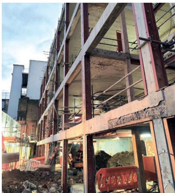
FIGURE 6: Existing concrete frame with steel strengthening
